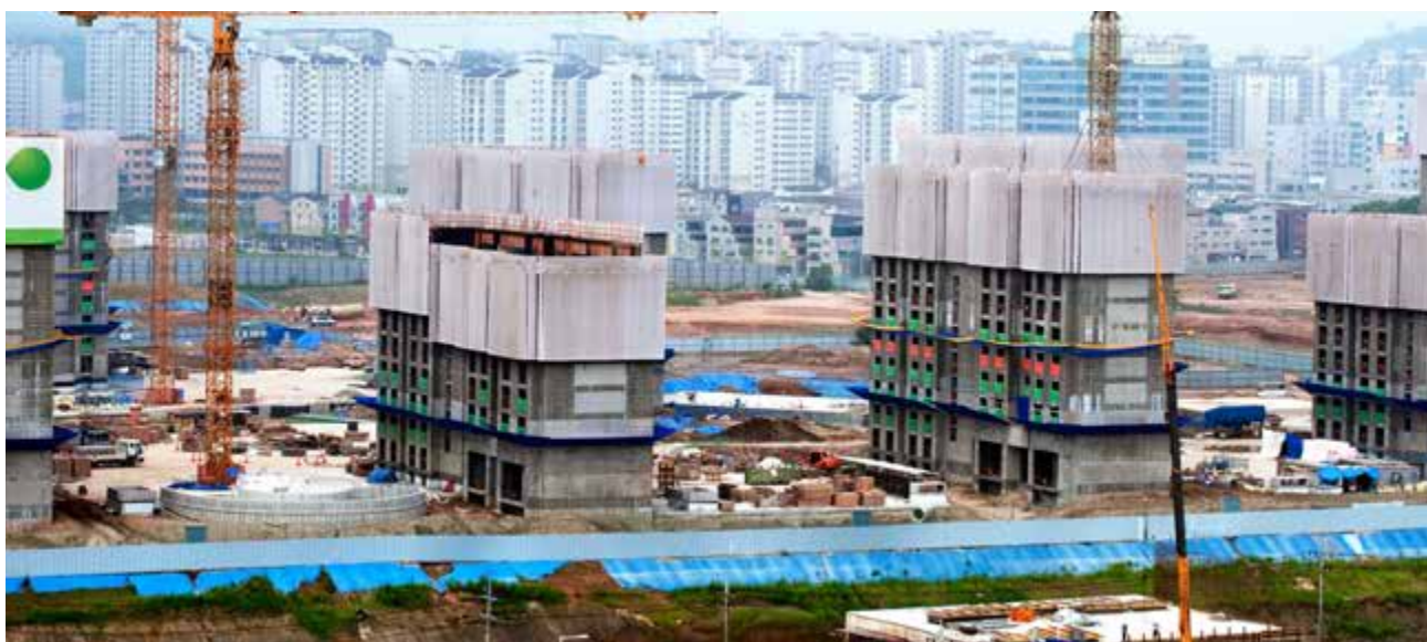
Construction sites in Busan, Republic of Korea © Kibae Park / ESCAP
